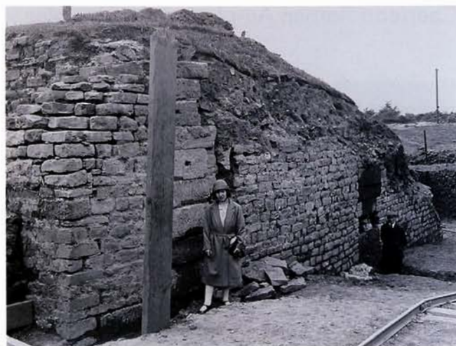
Mrs T. V. Wheeler standing in entrance B of the amphitheatre during its excavation
